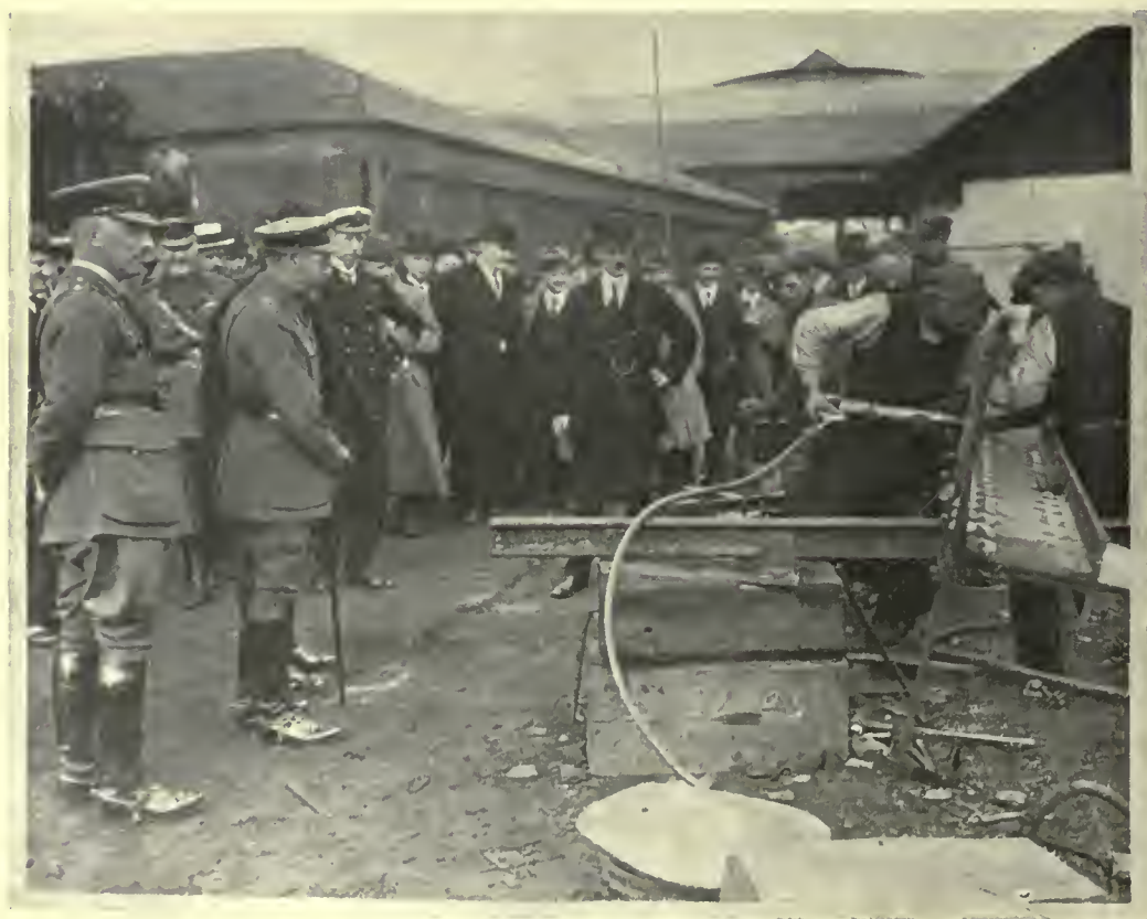
THE KING'S VISIT TO THE CLYDE, SEPTEMBER 18-21, 1917: WATCHING THE OPERATION OF A RIVETING MACHINE.
