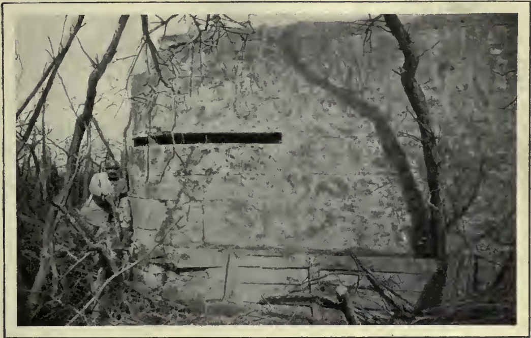
GERMAN CONCRETE "PILL-BOX" IN FLANDERS, WITH NARROW HORIZONTAL LOOP-HOLE GIVING A WIDE FIELD OF FIRE.
