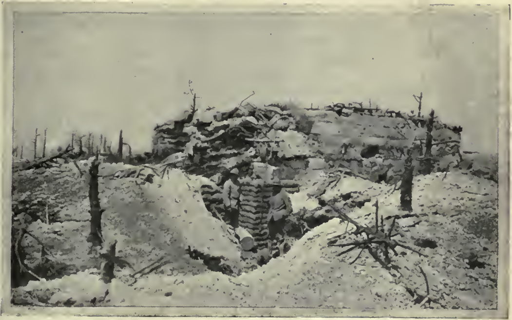
A GERMAN "BLOCKHAUS" ON THE CREST OF THE TÊTON.
