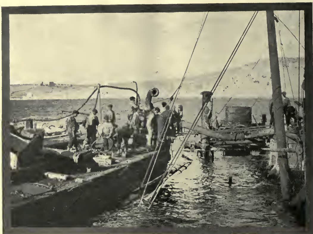
SALVAGE WORK ON A TORPEDOED STEAMER: RIGGING A PUMP.
