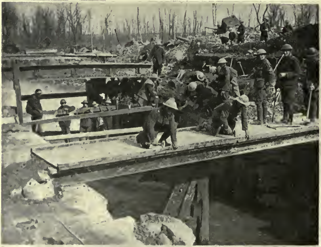
REPAIRING A LOCK.
