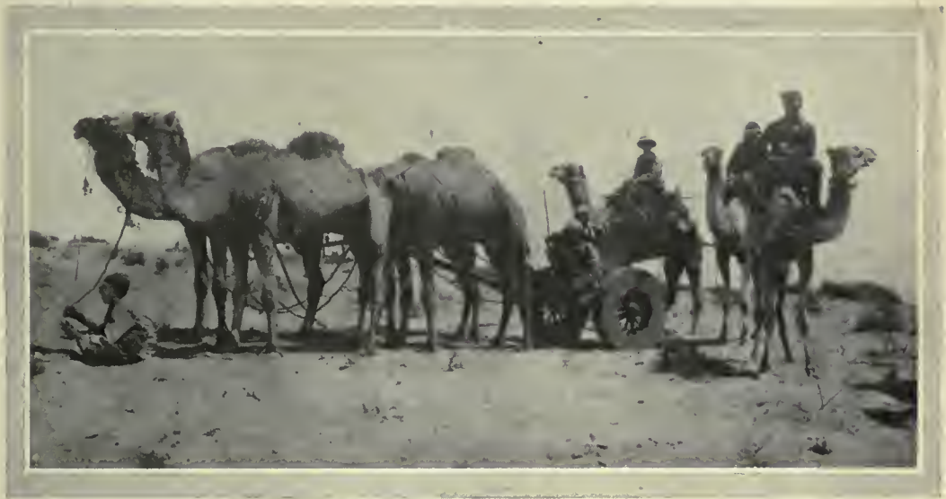
CAMEL TEAM DRAWING A CABLE-LAYING CHARIOT.
