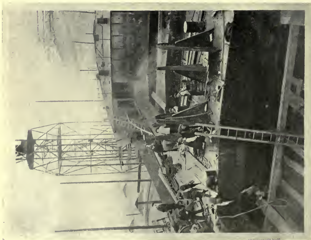
STANDARD SHIPS: ERECTING DECK FITTINGS.
