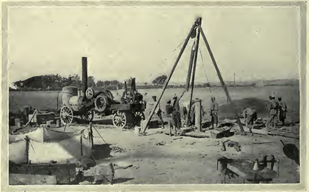
ENGINEERS BORING FOR WATER.
