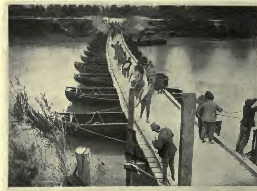
A PONTOON BRIDGE ON THE ISONZO.
