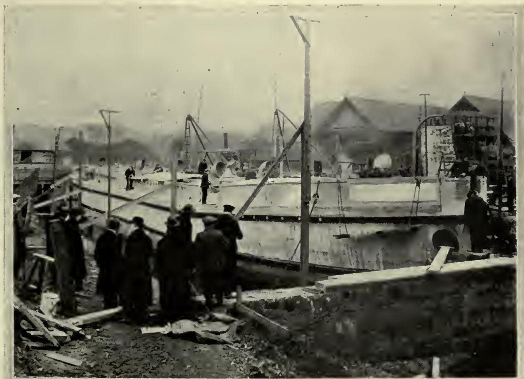
A CONCRETE SHIP NEARING COMPLETION.
